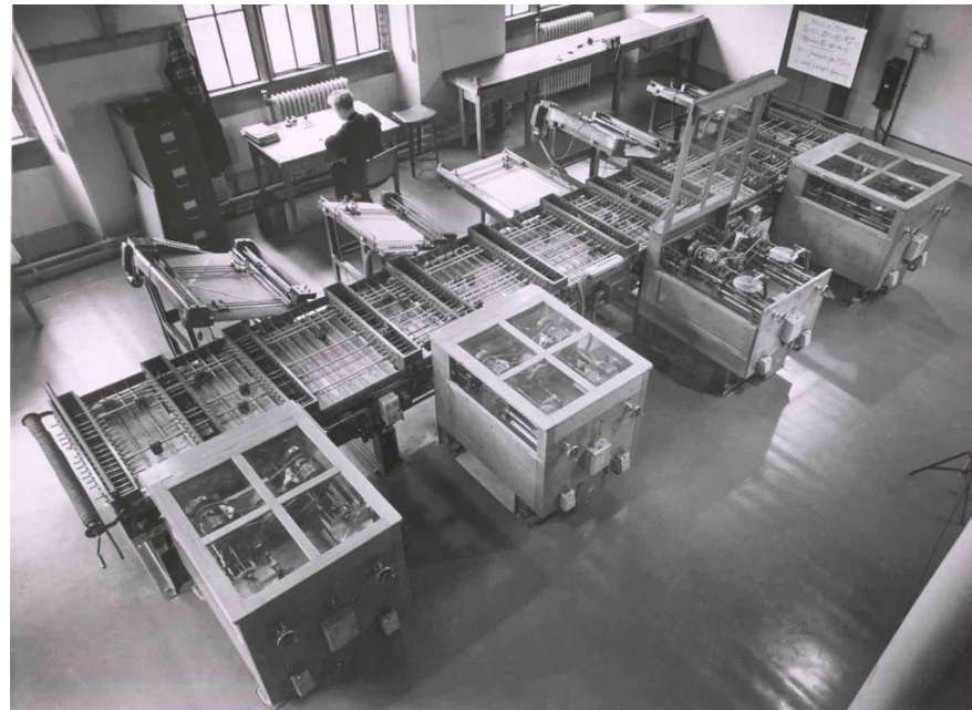
Differential Analyser, 1938, zdroj: University of Cambridge
